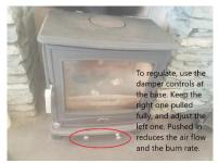
when adding fuel wait until the burn has died down significantly and rake it to make sure nothing will fall out when you open the door. Use the insulation glove provided to open the door and to add a log ,or add the coal from the scuttle or shovel. DO NOT TOUCH ANY PART OF THE STOVE WHEN IT IS HOT.
