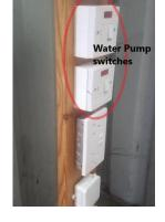
• If this fault cannot be reset, swap over the pumps by switching one off and the other on. BOTH PUMPS MUST NOT BE ON AT THE SAME TIME.
