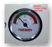
To run the heating or hot water, the water pump must be powered, and the pressure in the boiler at or above 1bar.
