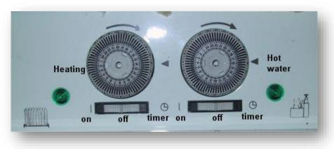
DON'T SWITCH ON THE HEATING OR HOT WATER IF THE PRESSURE IS NOT BETWEEN 1 AND 2.0 BAR..
